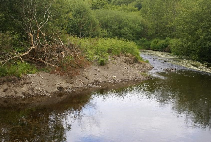
3: Dredging and bank works at Site FPM2 upstream
